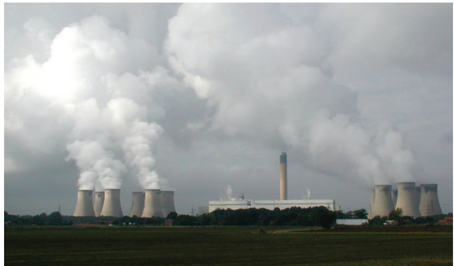
Drax power station (CC)
