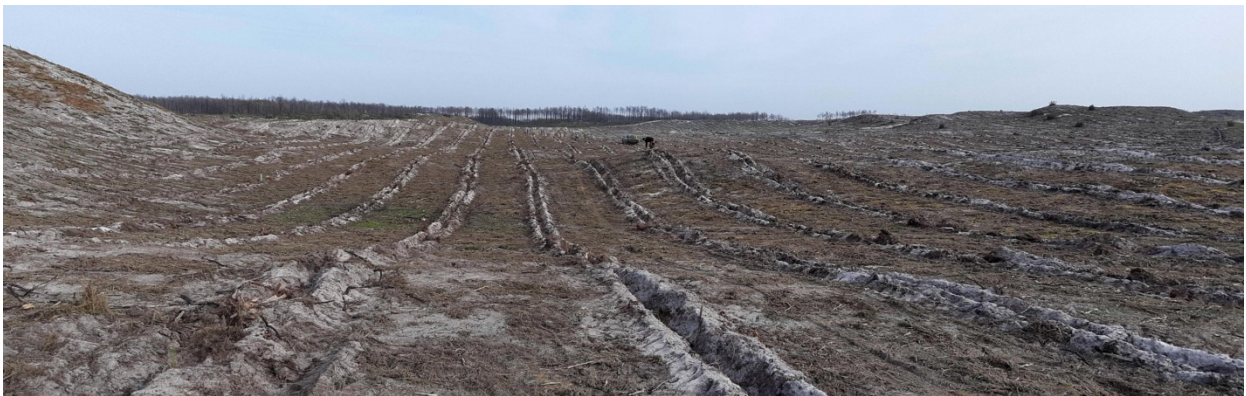
Parcel P3 after the preparation of the site.
